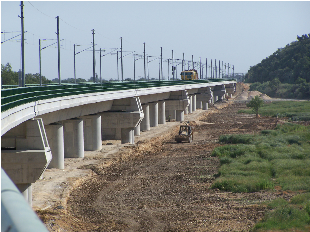
Figure 1: Santana do Cartaxo viaduct.
