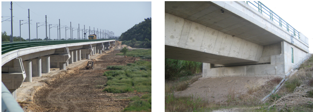
Figure 1: Santana do Cartaxo viaduct: general view (left); embankment (right)
