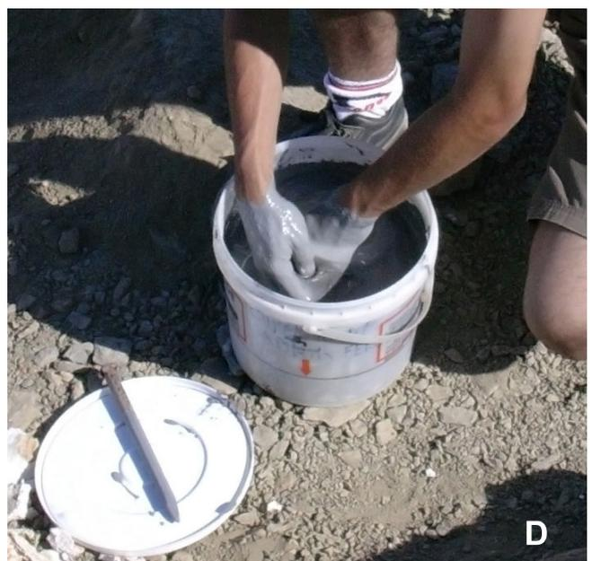
Fig. 1 – Procedure to use expansive cement: A- drill the holes using a hammer drill; B- transfer the expansive demolition agent to a clean bucket; C- mix homogeneously with the same proportion of water; D- pour the expansive cement in the drill holes previously opened.
