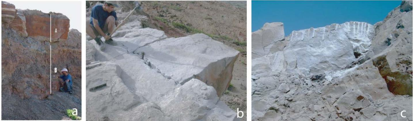
Fig. 2 – (a) Aspect of the sandstone layer A, above the bone-bearing layer B. Main block removed with combined technique stone-splitters and expansive cement, viewed from (b) top before removal, and (c) side after removal (drill holes still visible).
