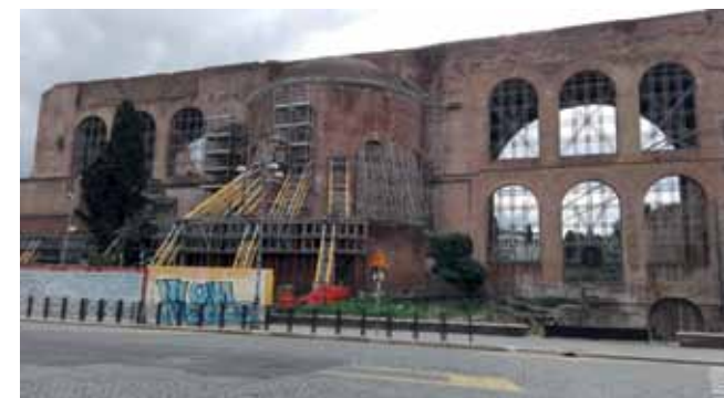
Figure 4.2. Reinforcement of Basilica of Emperor Massenzio along via dei Fori Imperiali during the construction of metro C in Rome, © L. Migliorati.
